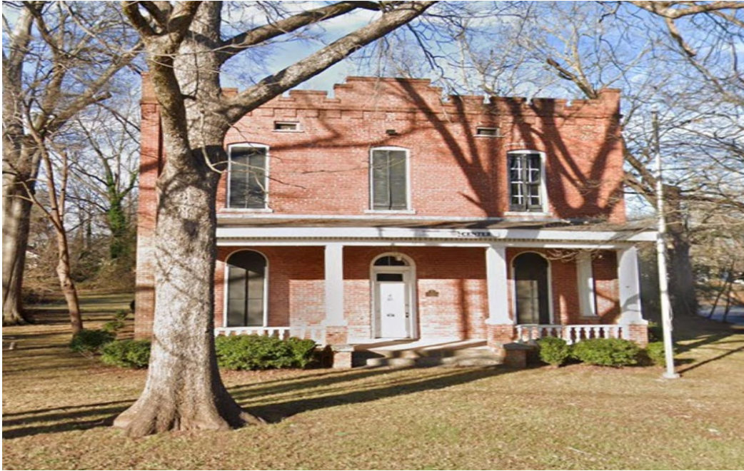
FIGURE 1:THE FIRST CLAYTON COUNTY JAIL BUILT IN 1869 LOCATED AT 125 KING STREET, JONESBORO, GA 30236.
